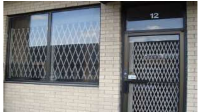
Storefront with folding security gates for window and door
